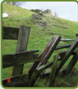
Broken stile or gate? No signs?
